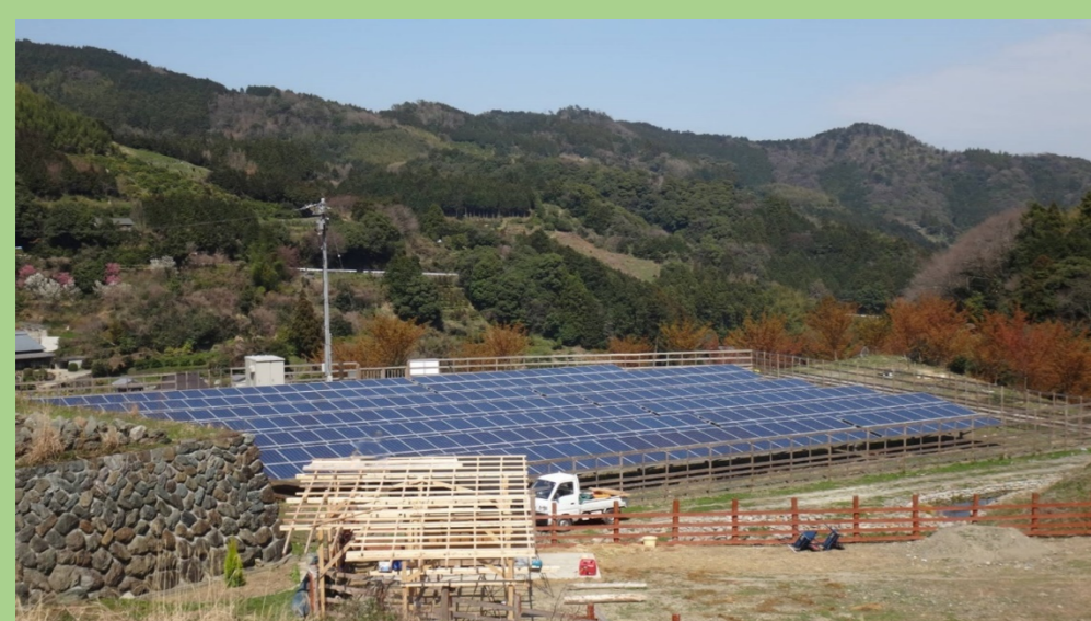
Community solar in Sanagochi Village, Tokushima
